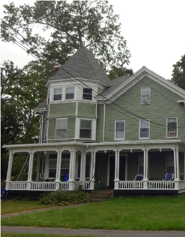
Existing 4-unit building in Newtonville.
