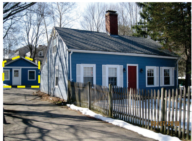
Image Source: Newton Inspectional Services Department
