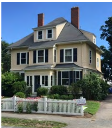
Left: Example of a pitched roof half-story
