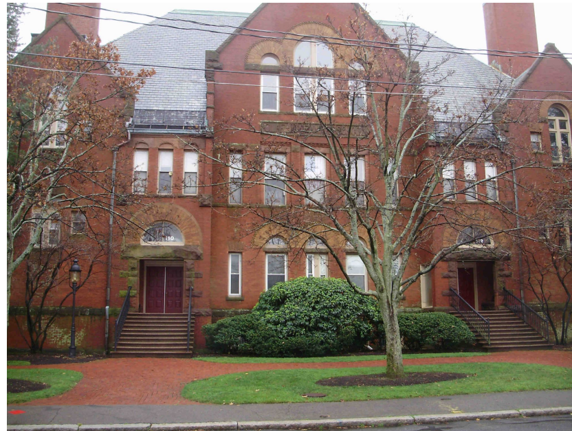
Clafin School Building - adaptive reuse and preservation
