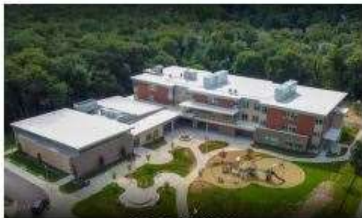
Green Buildings: Zervas Elementary School
