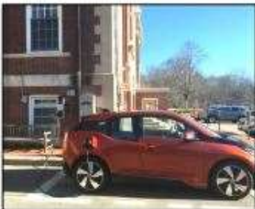
Clean vehicles: City Hall EV charging station
