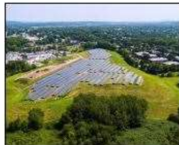
Renewable Energy: Solar array at Rumford Avenue
